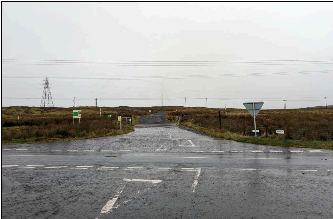
Access into the Inverclyde Wind Farm taken from the B788
