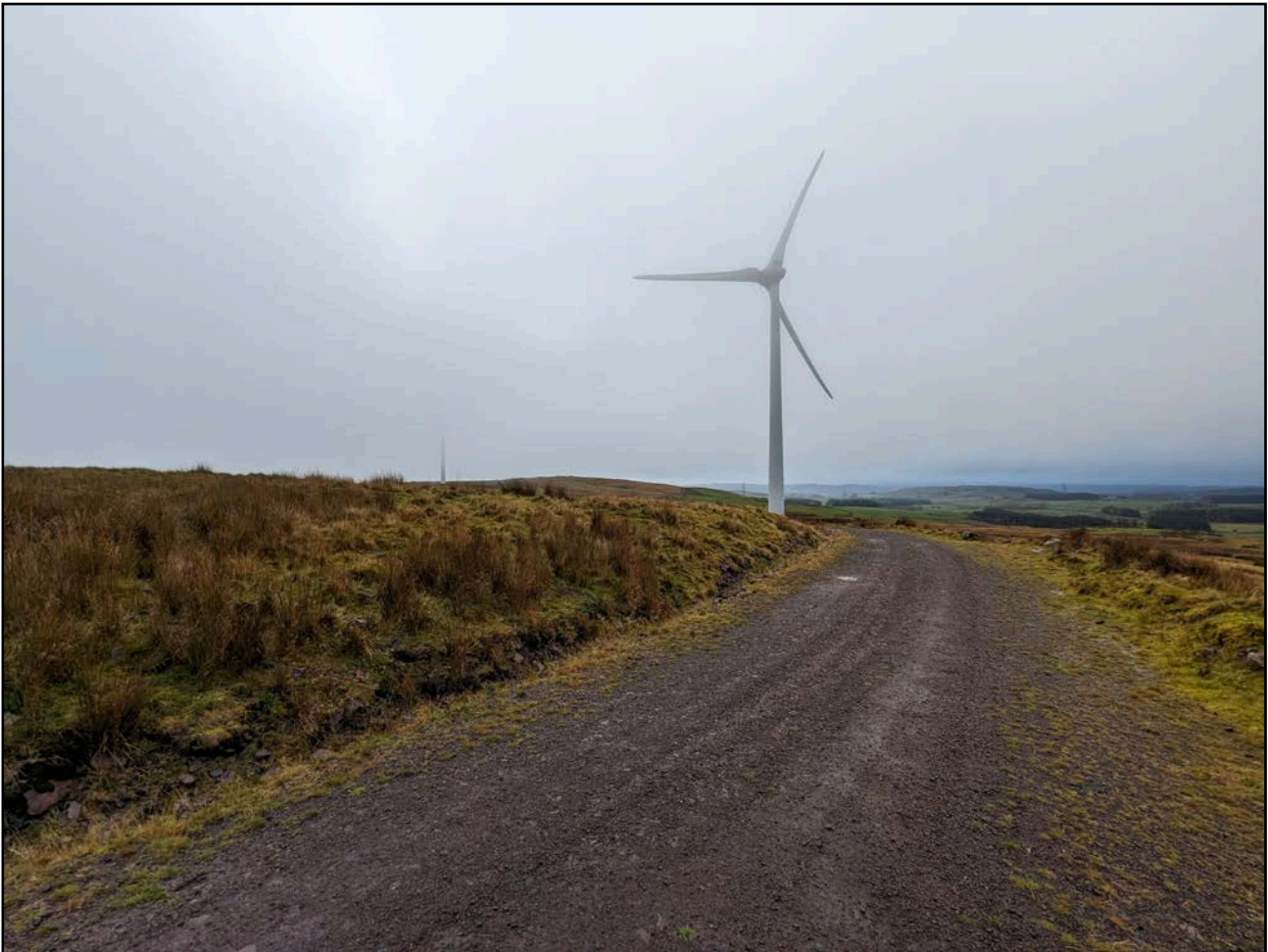
Interior of site: track and turbine facing north west into the site
